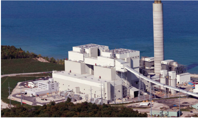
Elm Road Generating Station
