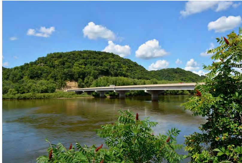
U.S. Highway 61 crosses the Lower Wisconsin River via the Boscobel Bridge. The bridge is dedicated to one of the city’s well-known residents,
