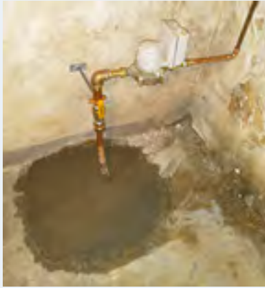
Basement in New Glarus after completing LSL replacement.
